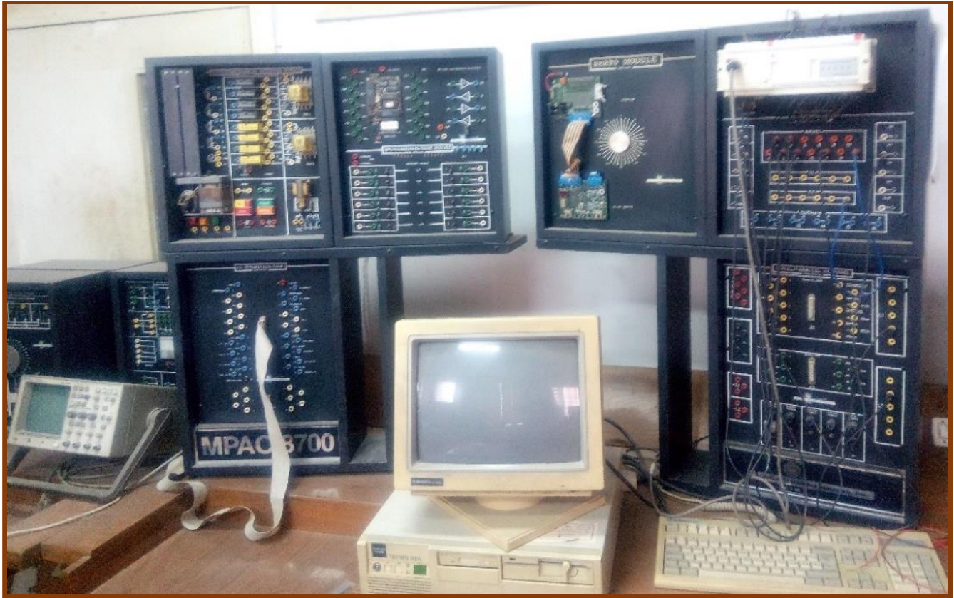
Programmable logic controller board 1
